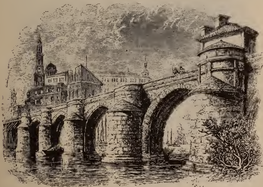
BRIDGE AT ZARAGOZA.
